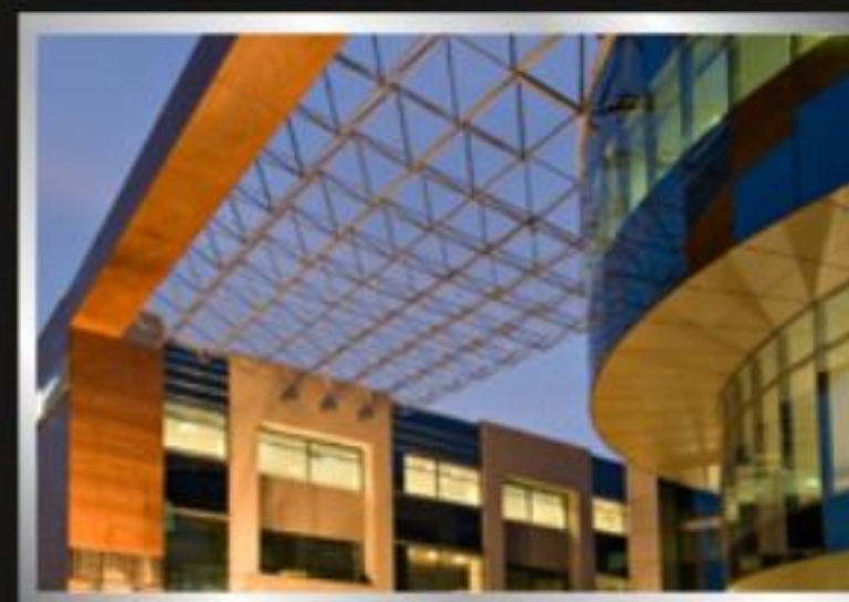
PATNI KNOWLEDGE CENTER, NOIDA (BLOCK B) GOLD RATED LEED CERTIFIED GREEN BUILDING - 2011
