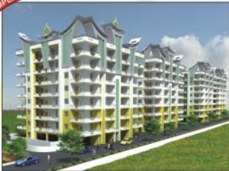
Amrapali Awadh, Lucknow
